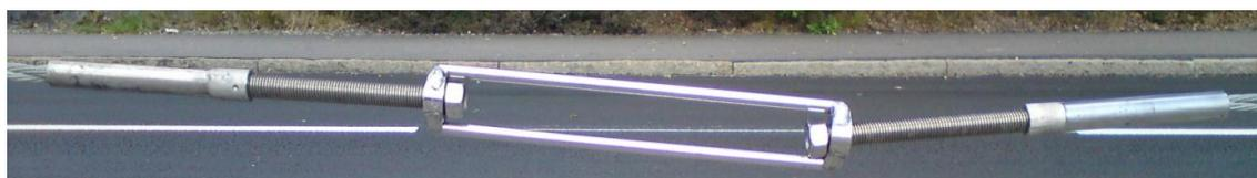
Picture 4. Install tensioning unit in cut gap.
